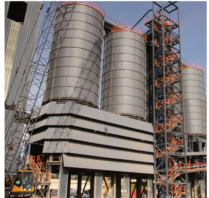
The latest state-of-the-art cement production factory at Namataba, Kampala. COURTESY PHOTO
